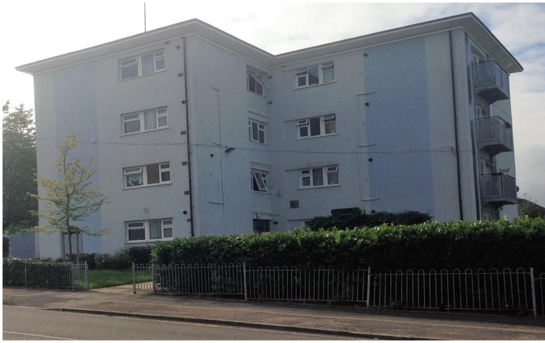
Refurbished flats on Robin Hood Avenue
